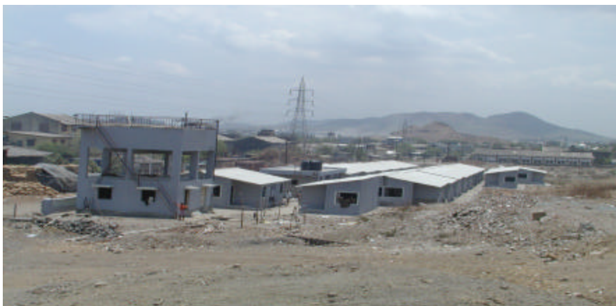
View of housing rehabilitation scheme under construction for slum dwellers
